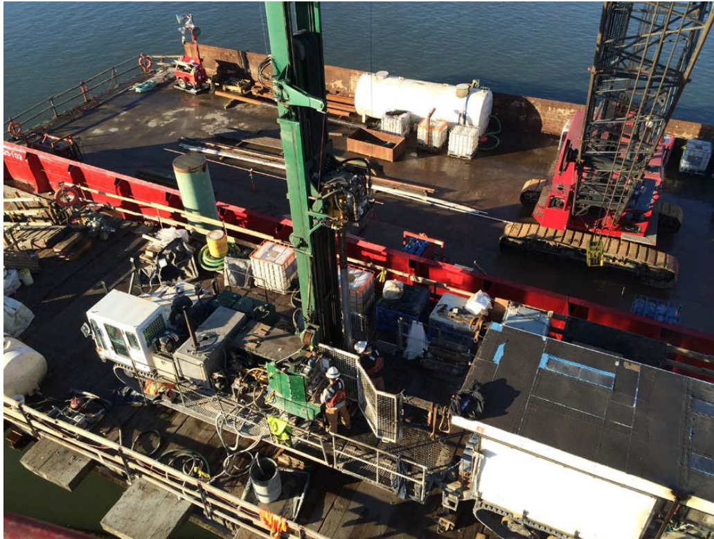
Figure 6. Freeze Pipe Drilling Operation
