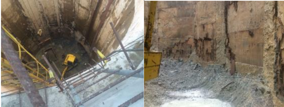
Figure 8. Inspection of slurry wall after pump down
