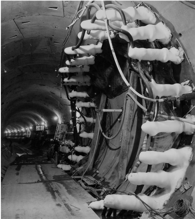
Figure 10. Ground freezing system CP-23.
