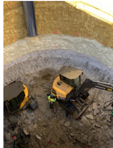
Figure 9. Excavation of Launching Shaft
