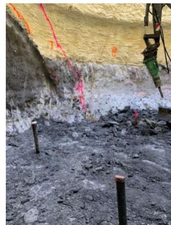
Figure 10. Completed Excavation with Abandoned Interior Pipes
