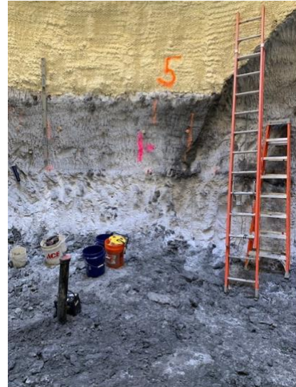
Figure 8. Application of Polyurethane Insulation
